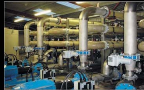
Biomass separation using crossflow ultrafiltration modules.
